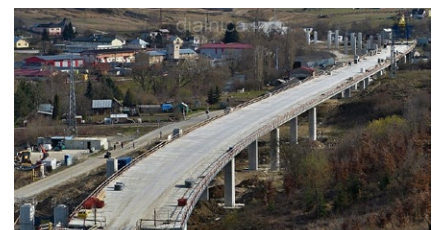
Impression from the bridge 209-00 construction close to Lietavská Lúčka village
