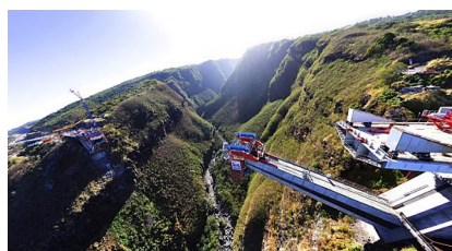
Bridge under construction
