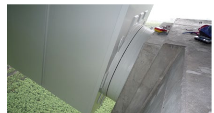
RESTON®POT load measuring and injection bearing with load capacity 60,000 kN
