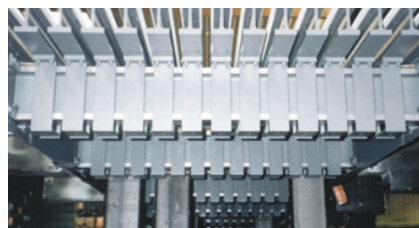
6 TENSA®MODULAR expansion joints 1,200 mm movement (LR15)
