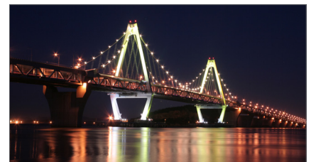
Night view of Yeongjong Grand Bridge
