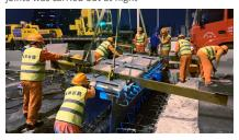
A TENSA®FINGER GF in its final position on the bridge
