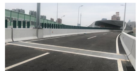
One of the installed TENZA®POLYFLEX®ADVANCED PU joints
