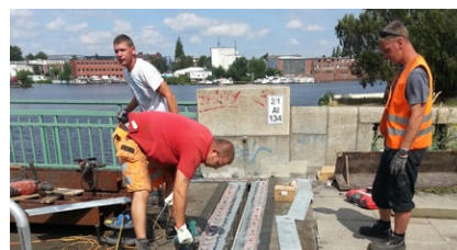
Section 1 and 2: Joint installation
