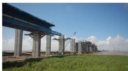
The Chong Ming Crossing during construction
