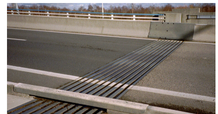
Modular joint preserves faultless functionality even in the case of a steep longitudinal slope (here 6%)
