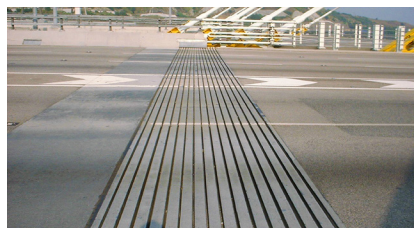
Modular joint type LR 16 with anti-skid surfacing
