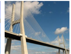
Vasco da Gama Bridge (포르투갈)
