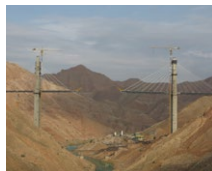
Lali Bridge (이란)
