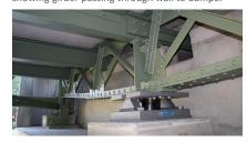
Seismic damper in access shaft, from above (connecting though wall on right to deck girder)
