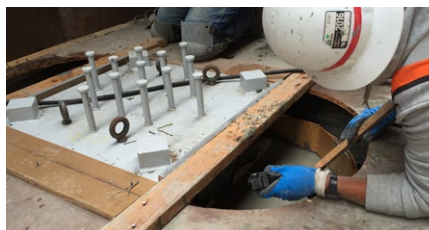
Installation of RESTON®PENDULUM Mono on terminal superstructure
