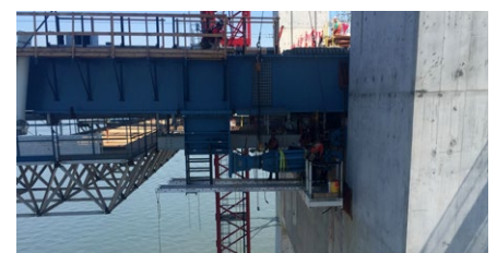
Installed shock transmission unit
