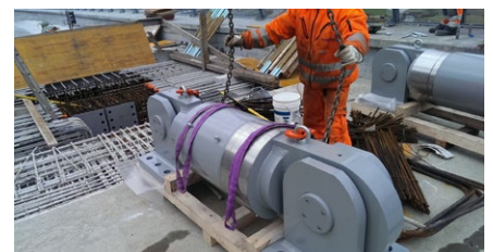
Installation of a RESTON®STU shock transmission unit in the viaduct's deck
