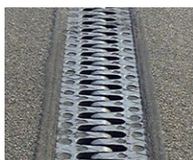
Cantilever finger joints
