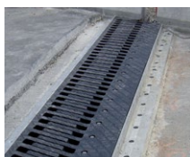
Sliding finger joints
