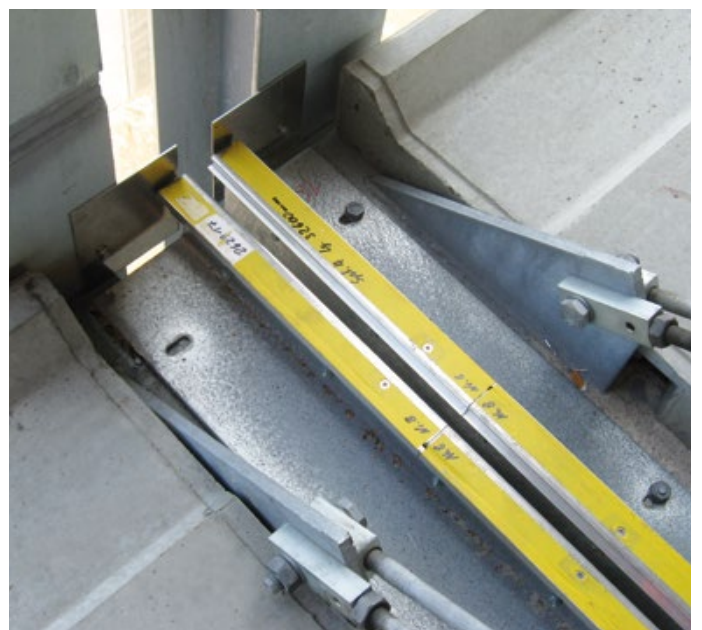
Parking garage Weiterstadt, Germany – FP 90
