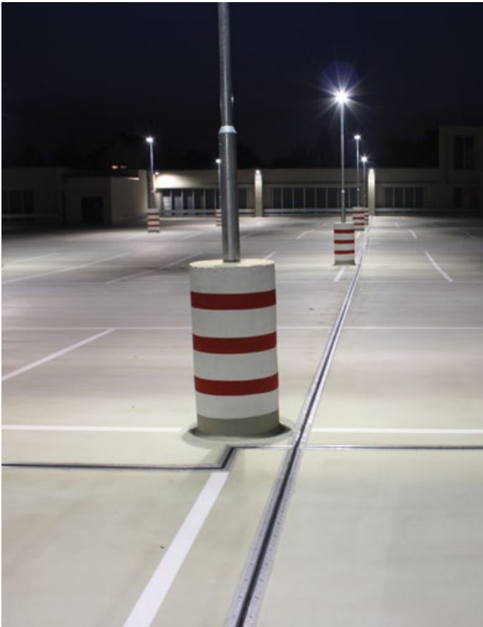
Parking deck shopping mall Dresden, Germany
