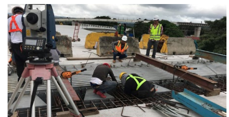
Leveling and fixing of TENSA®MODULAR to reinforcement rebars before concrete casting
