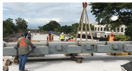
Modular joint handling with help of a crane
