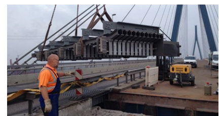
Incorporation of the new waterproof noise-relieved expansion joints
