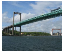
Alvsborg Bridge (SE)
