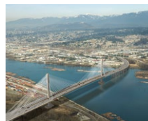
Port Mann Bridge (CA)
