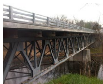
Route 9G Bridge, NY (US)
