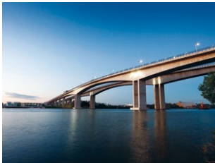
Puente Gateway, Australia
