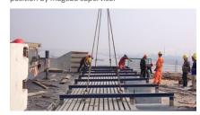
Impression from the construction site: preparation of concrete works for the expansion joints
