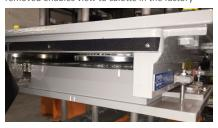
Installed RESTON®SPHERICAL bearing
