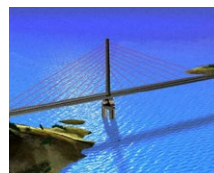
Agin Bridge (TR)
