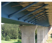
Ponte Steinbachtal (DE)
