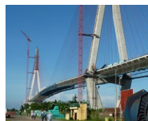
Ponte Can Tho (VN)
