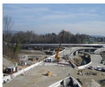
Ponte Sihl (CH)
