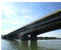
Ponte Traismauer (AT)
