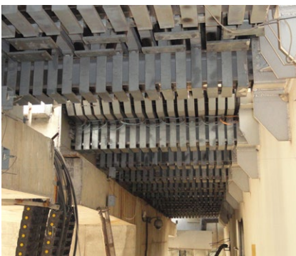
Expansion joints with sensors installed
