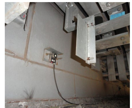
Ultrasonic sensors installed on the joint
