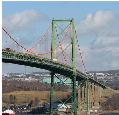
Angus L. Macdonald Bridge
