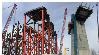
Erection of the cable stay bridge
