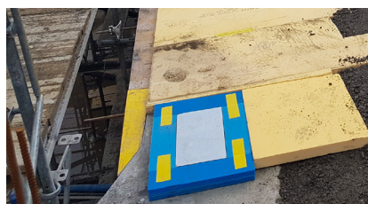
Installation of the LASTO®FLONPAD GA-C bearings on the wall crown
