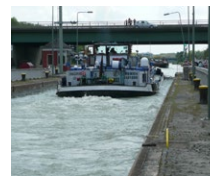
Hindenburg Bridge (DE)
