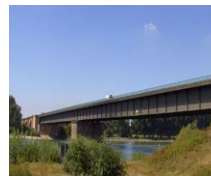
Rhine Bridge Frankenthal (DE)
