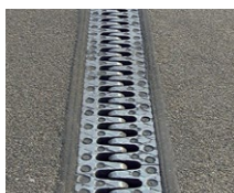
Cantilever finger joint
