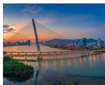
Tran Thi Ly Bridge (VN)
