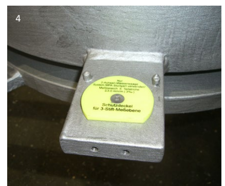
1 Anchor studs on anchor plate 2 ROBO®SLIDE 75 sliding material 3 Application of lubricating grease 4 Optional console for 3-point levelling surface
