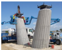
Santa Maria Bridge (ES)
