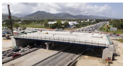
Construction of one of the new bridges
