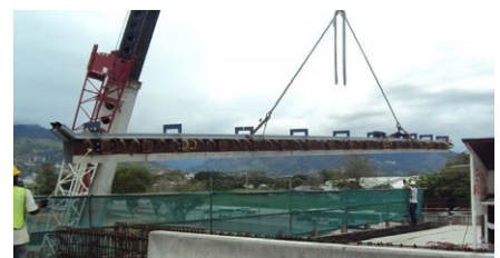
Installation of a mageba TENSA-MODULAR LR2 expansion joint
