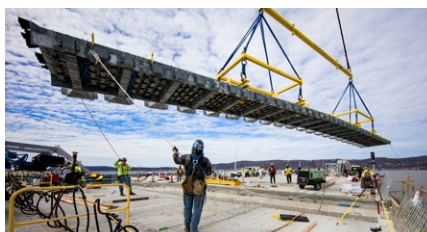
Installation of a TENSA®MODULAR expansion joint type LR8
