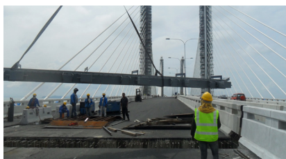
mageba Tensa®MODULAR expansion joint of type LR 5 during installation
