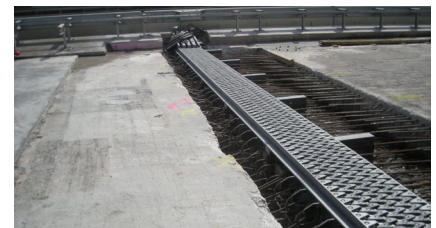
Installation of a TENSA®MODULAR expansion joint (type LR4-LS100), prior to concreting
