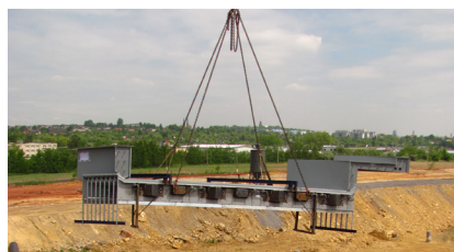
Lifting of a TENSA®MODULAR type LR8-RW joint into position on the bridge
