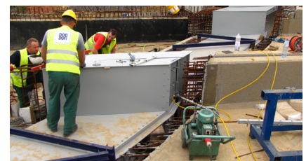
A TENSA®MODULAR joint of type LR8-RW (railway bridge joint) during installation
