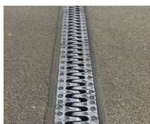
Cantilever finger joints
