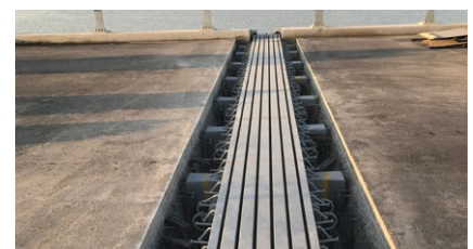
A TENSA®MODULAR LR6 joint in its recess
