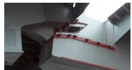
Support points of the finger lock
