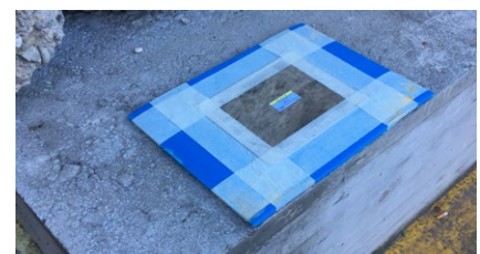
Bearing before concreting view from below
