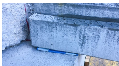
Bearing before concreting view from above
