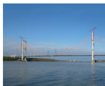
Audubon Bridge (USA)
