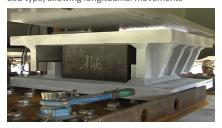
Lead rubber bearing installed in the bridge – multi-directional type, allowing all movements
