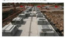
A typical RESTON®FORCE horizontal force guided bearing – resisting only transverse forces
