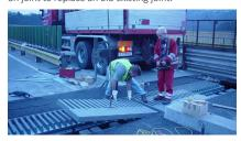
A TENSA®FINGER sliding finger expansion joint (type GF600) as installed, work almost complete.
