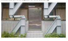
Close-up view of a RESTON®SA shock absorber, as installed
