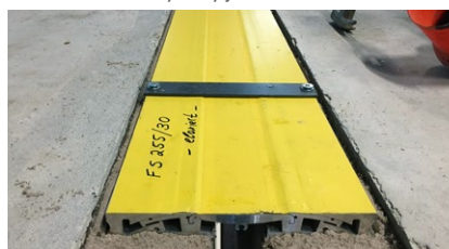
MIGUTRANS heavy-duty joint laid in a mortar bed
