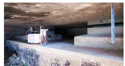
Measuring equipment on the abutment
