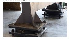
Construction of the anaerobic digester on top of the installed LRBs
